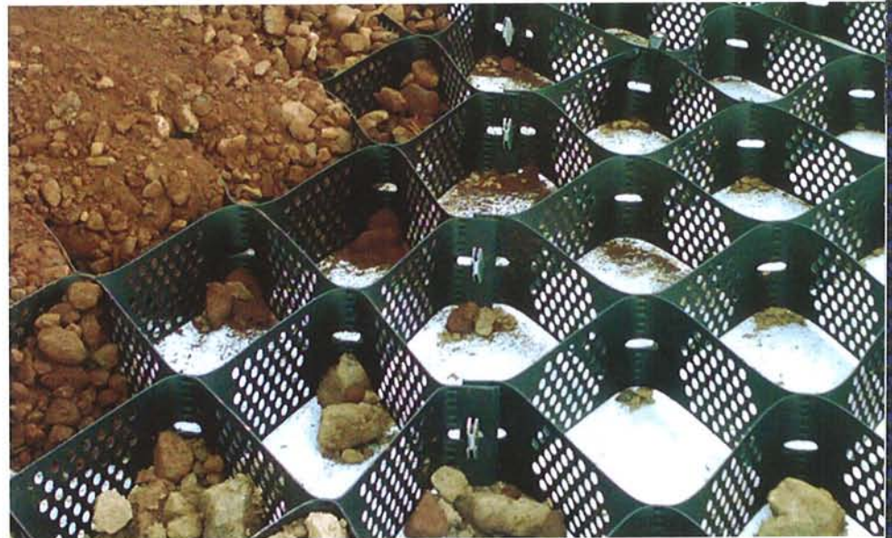
FIGURE 4 Expanded and connected geocell sections partially infilled
