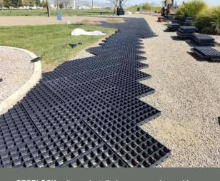
GEOBLOCK units are installed over an engineered base in a herringbone pattern for multi-directional traffic.
