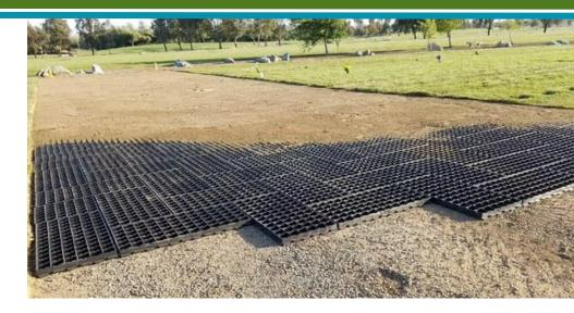
GEOBLOCK®5150 grass porous pavements were designed for frequent traffic with H-15 loading.
