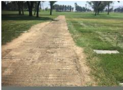
Top photo: An engineered base (aggregate/topsoil mix) is placed.
